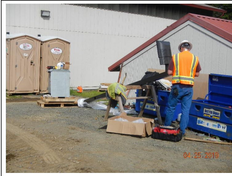
Assembling the outdoor over head light poles for the SBR.
