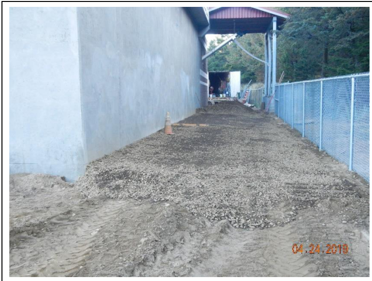
Grading truck loading access road.
