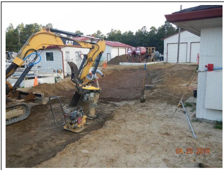
Setting digester access road subgrade
