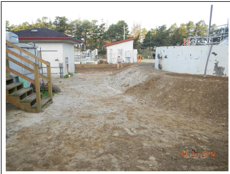
Final surface grade around digester 5.
