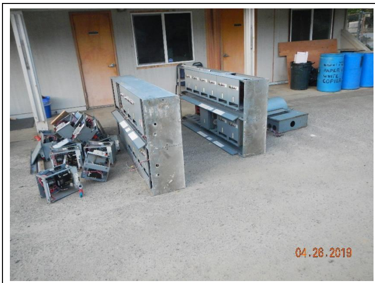
Completed removing the remaining electrical equipment from the administration building.
