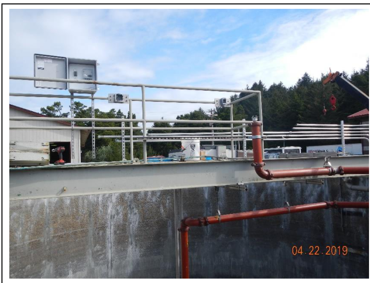
Installing electrical conduits and pulling wires to digester 5 equipment.
