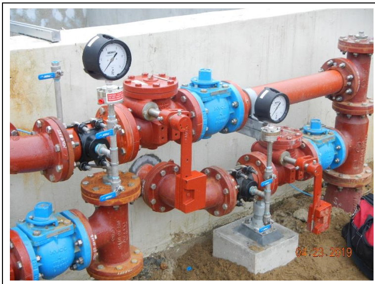
Installing pressure gauges on the FHT pump piping.
