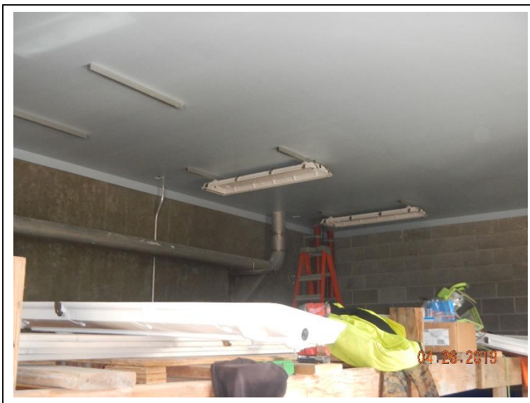
Installing the blower room ceiling lights.
