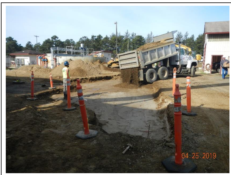
Bringing in gravel to finish SBR access road subgrade.
