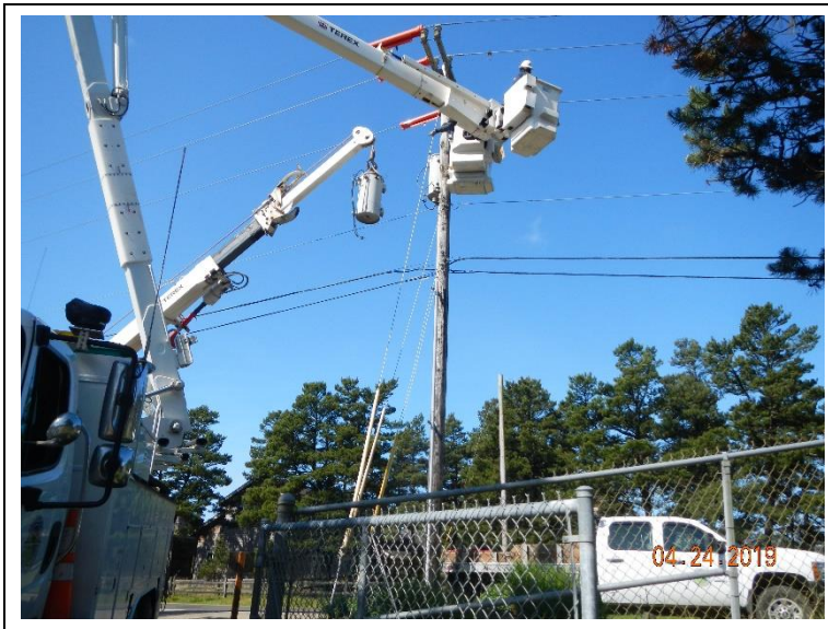
Tillamook PUC removing transformers that provided power to the site.
