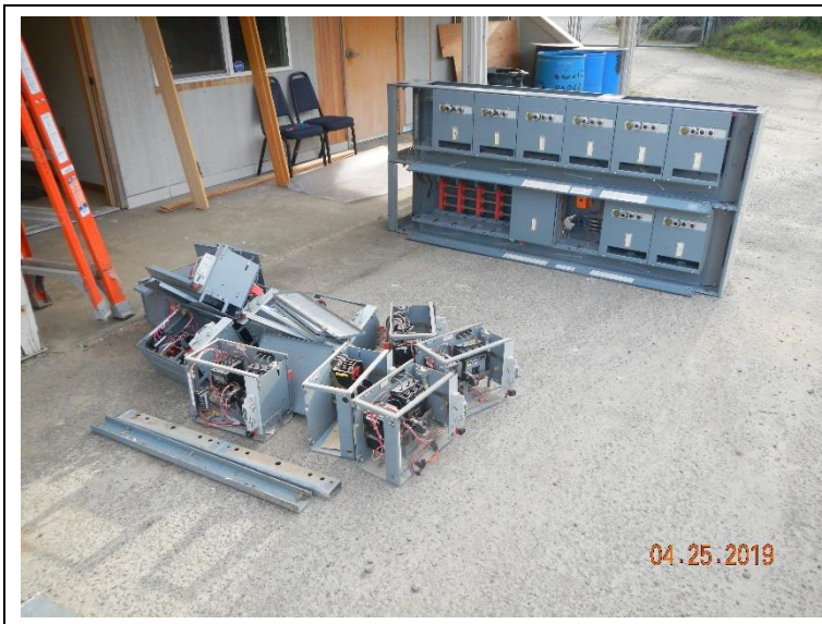
Removing the old electrical equipment from the administration building.
