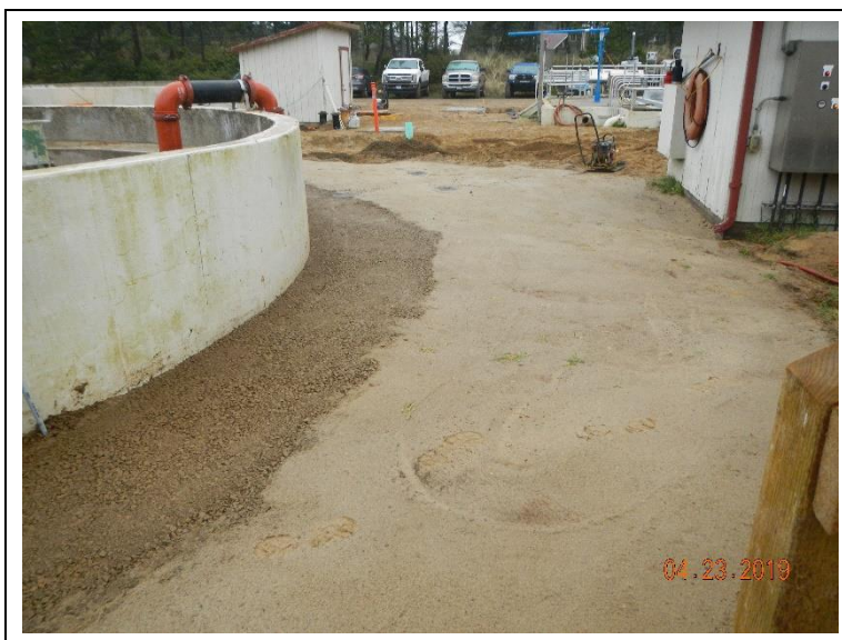
Setting finish surface grade around digester 4.
