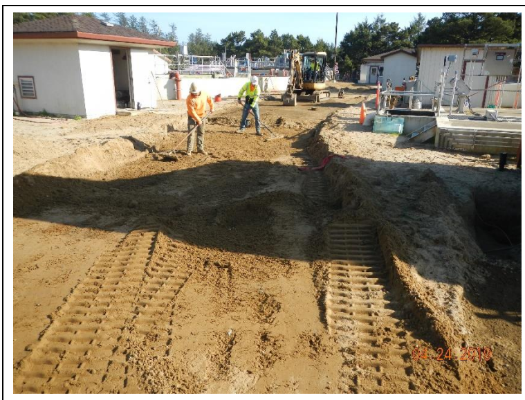
Preparing digester access road subgrade.
