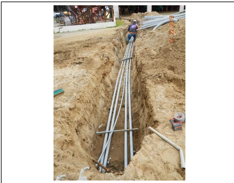
Installing electrical conduits from UV generator building to the maintenance shop.
