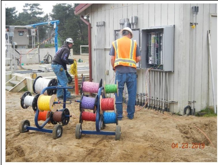
Pulling wires to the reuse water motorized butterfly valve.
