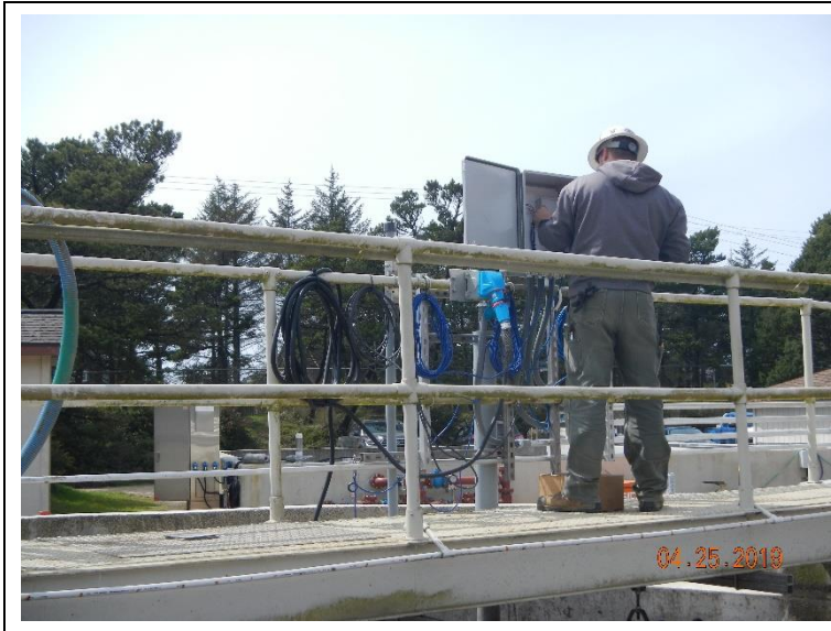
Completing the electrical wiring to digester 3.
