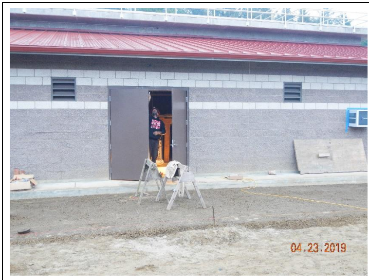
Installing blower room double doors.
