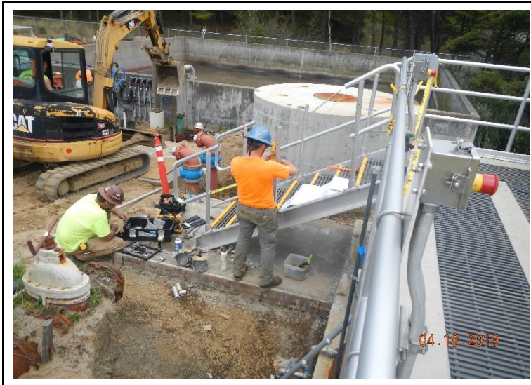
Installing the northside stairs and hand rails at the headworks.
