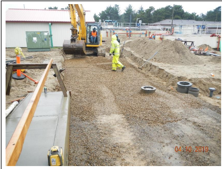
Placing subgrade rock for SBR access road.
