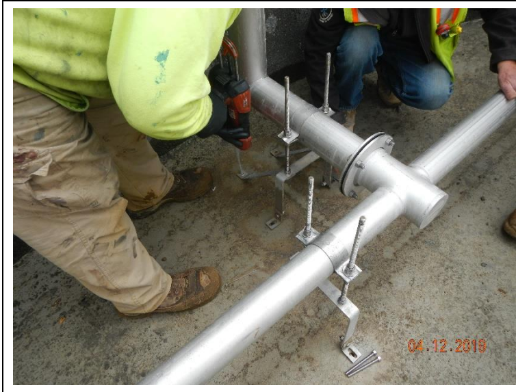
Setting epoxy anchor bolts on digester 5 air diffuser piping supports.
