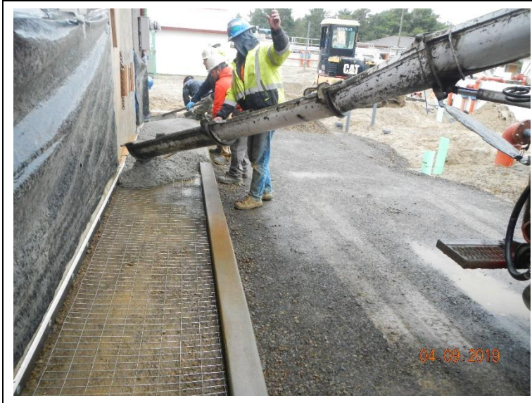
Pouring concrete for SBR sidewalk.
