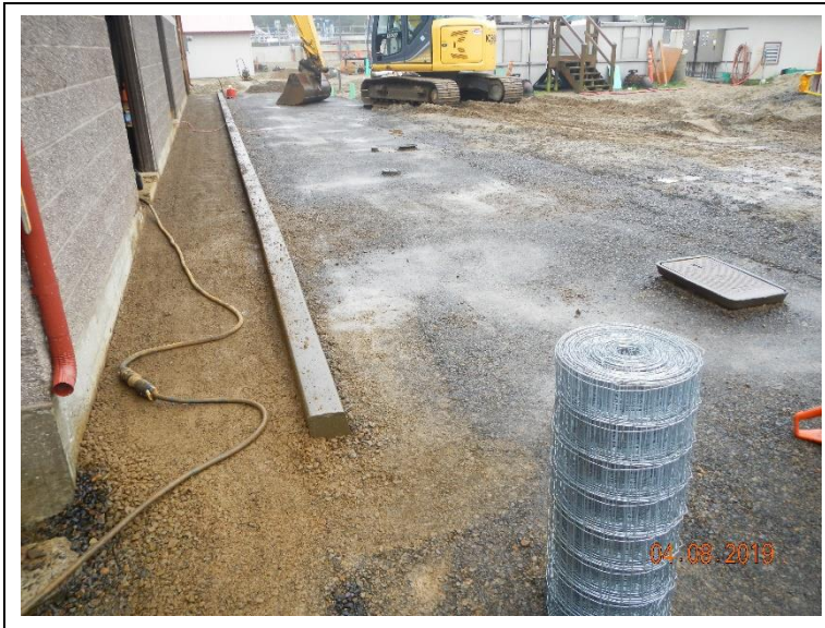
Completed backfilling sidewalk subgrade.
