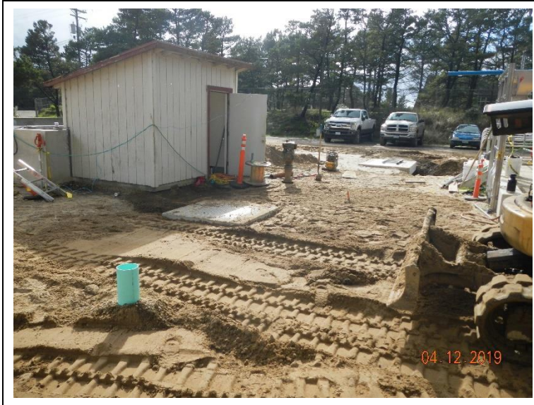
Backfilling around the reuse water vaults.
