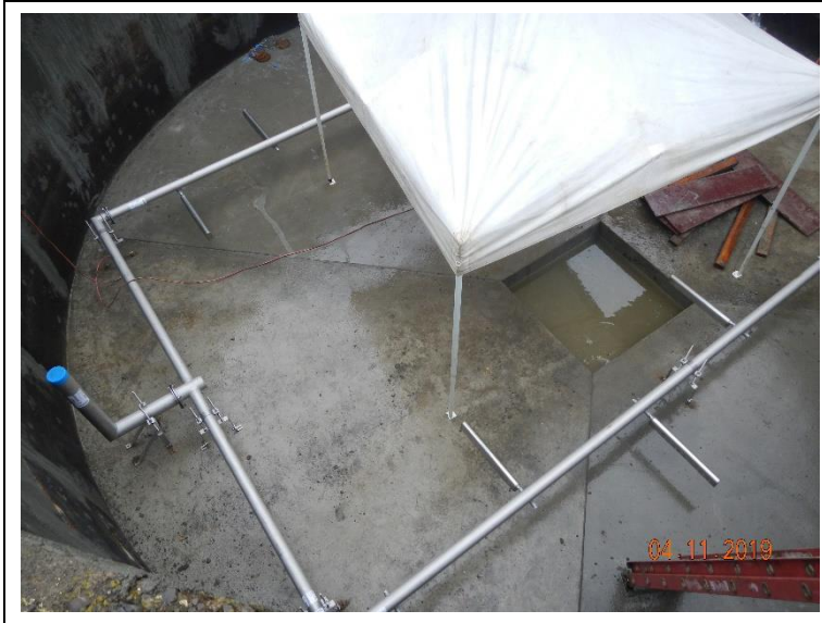
Installed the air diffuser piping in digester 5.
