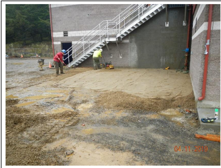
Setting surface grade at the northwest corner of the SBR
