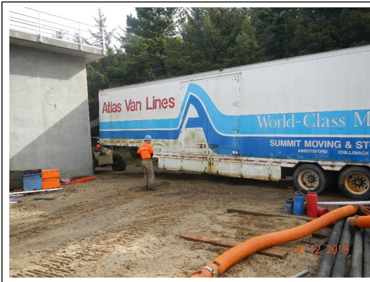
Moving the equipment storage trailer and beginning to clean-up the site.
