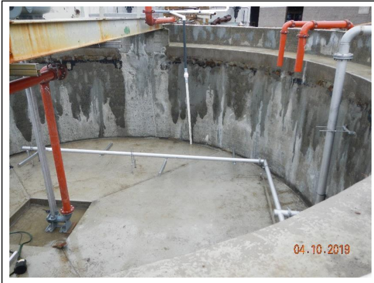
Installed the air diffuser piping and supports in digester 5.
