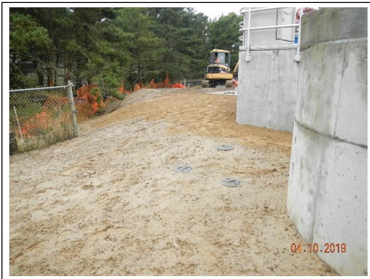
Setting surface grade around the headworks.
