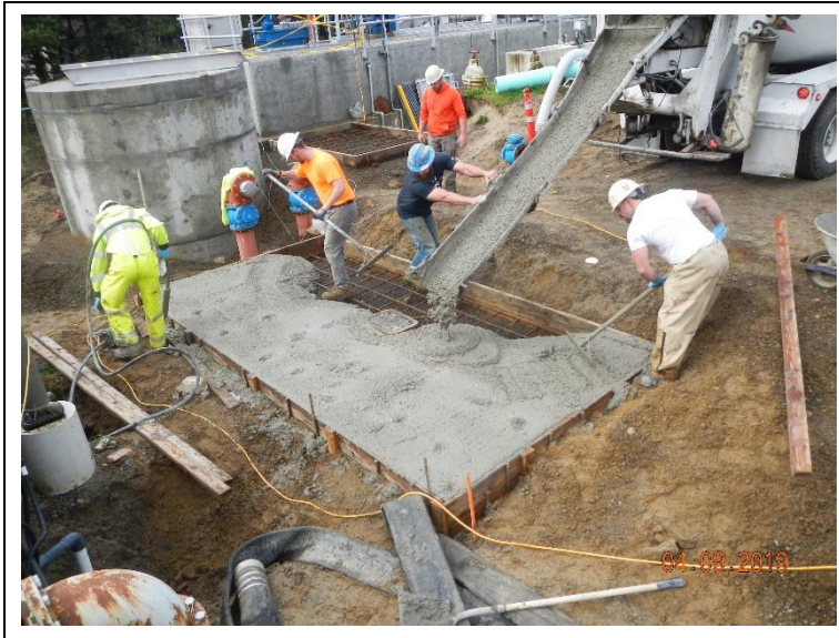
Pouring concrete for FEB bypass pump slab.
