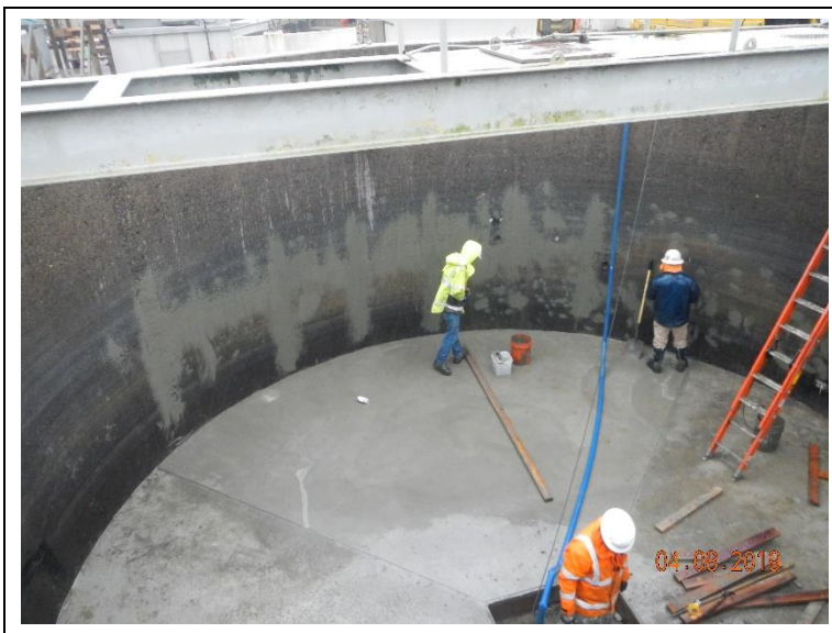
Grout patching digester 5 walls.
