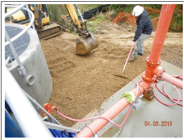
Setting surface grade around headworks grit chamber.
