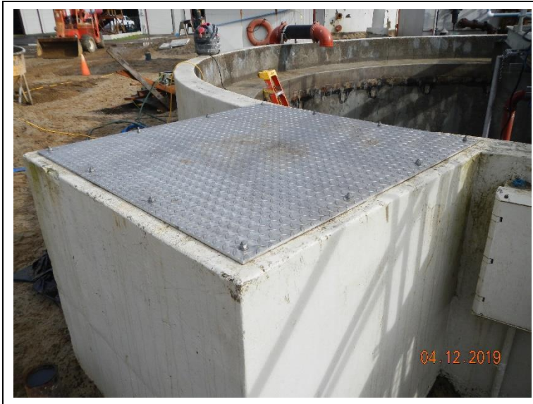
Installed aluminum plates over the sludge wells on digesters 3&4.
