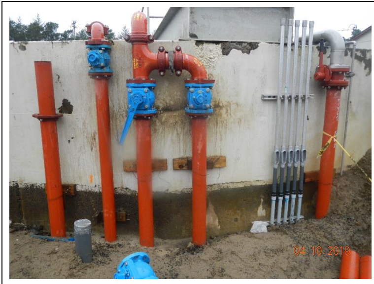
Installing the WAS, DR and DS piping into digester 5.
