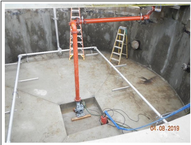
Installing aeration diffuser piping and WAS pump piping in digester 4.
