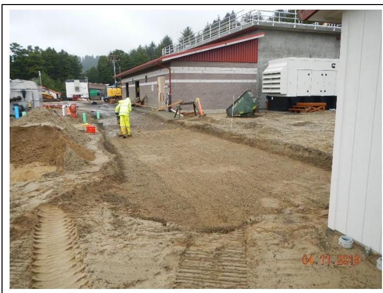
backfilling SBR access road and setting subgrade.
