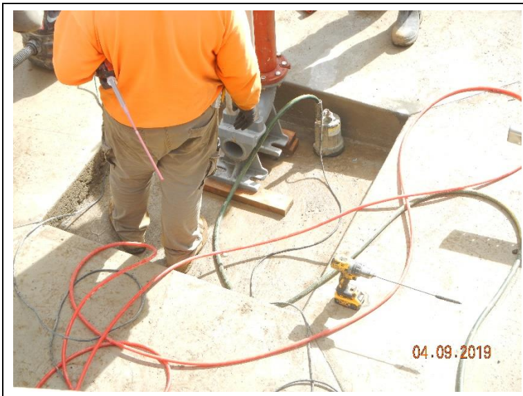
Setting epoxy anchor bolts for WAS pump base in digester 4.
