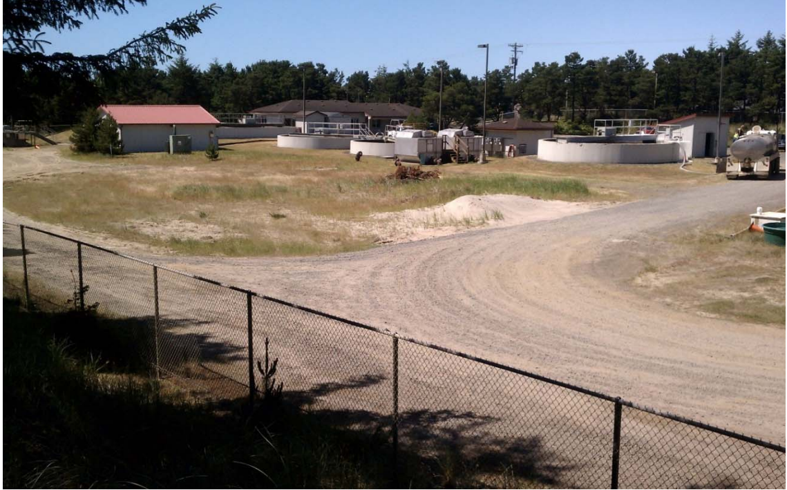
Photograph 3. Project area; looking southwest from eastern boundary.
