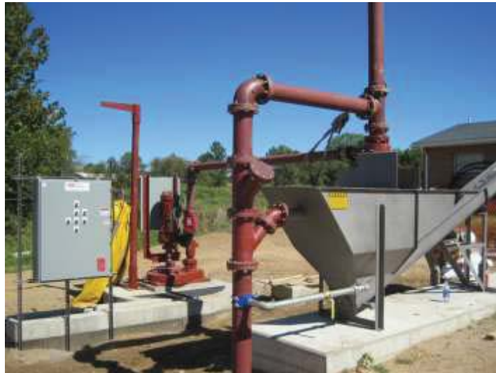
Complete PISTA® Grit Removal System Installation Photo
