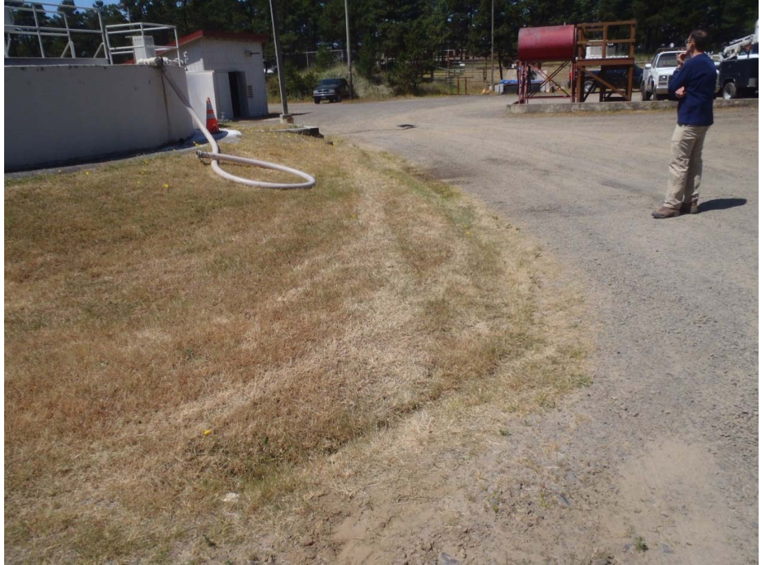
Photograph 7. Stormwater inlet area.
