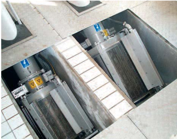
ROTAMAT® Rotary Drum Fine Screens Ro 2, directly installed in channels; available with basket diameters from 2 to 10 ft (0.6 to 3 m)
