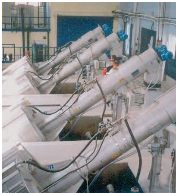
Four ROTAMAT® Rotary Drum Fine Screens provided with integrated screenings washing (IRGA)
